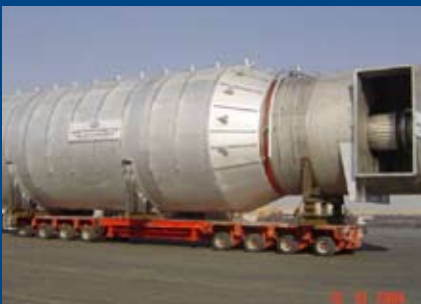
Thermal Oxidizer 6.4m diameter x 15m long GACIC BDO Facility, Sipchem
