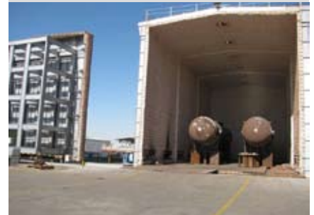
▶ PWHT Furnace Capacity: 30m Long x 13m Height x 13m Width
