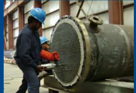
HP Cooler 0.7m diameter x 6m long Yanbu Petrochemical Complex, Sabic
